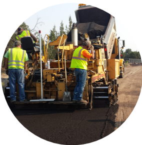
Street Repair & Maintenance
